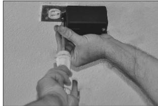
**B) Two screws securing cover plate, one on top and bottom:**
