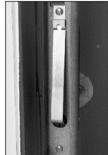
9. At this point check and confirm that SureLock's Lock-Bar(C) movement through track is clear and smooth. You will need to shift the Red Release Lever towards the track (Locked Position). With SureLock in normal operating position simply depress the Lock-Bar(C) from inside of track with your hand a few times to ensure smooth / clear operation.
